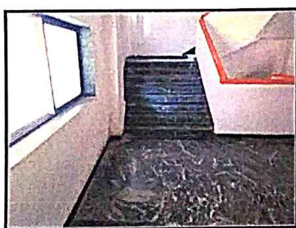
Daylight at Staircase
